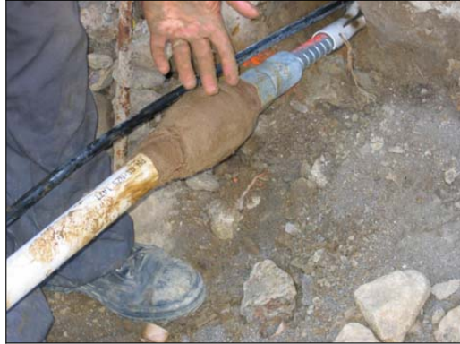
Figure 7: PVC & Denso in unbonded area
