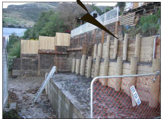
Figure 9: Completed wall from side
