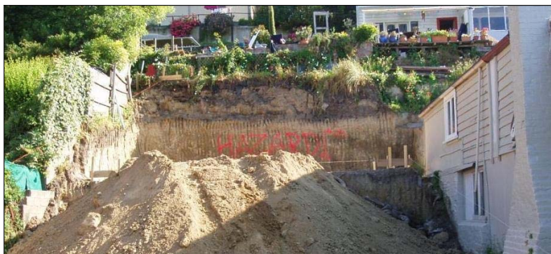
Figure 2: Excavation as at the end of December 2004
