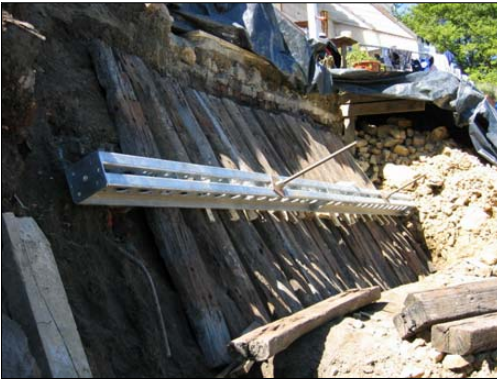
Figure 8: Temporary stability works
