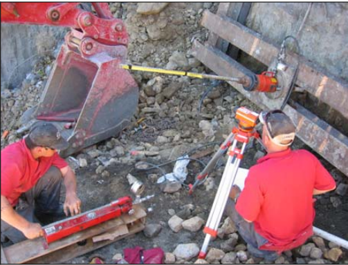
Figure 6: Testing Anchors
