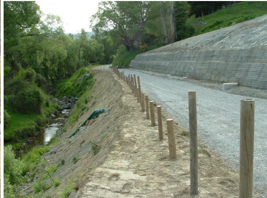
Figure 11. Otaihape remedial works
