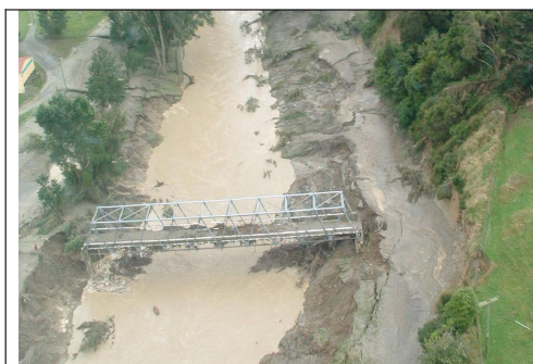
Figure 3. Aerial photo of McLays Bridge.
