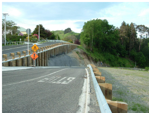
Figure 13. Papakai Road remedial works
