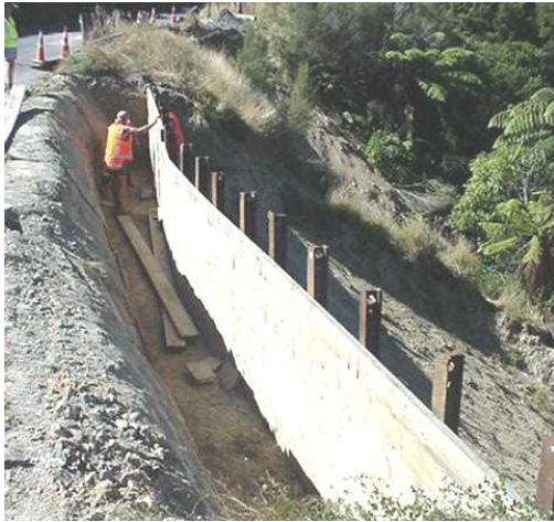
Figure 9. Railway Iron Retaining Walls Rangiwahia Rd
