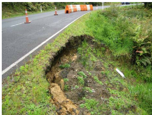
Figure 4: Photo showing failed portion of Murray Road
