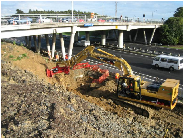
Figure 3: Photo showing installation of LSNs into bridge embankment
