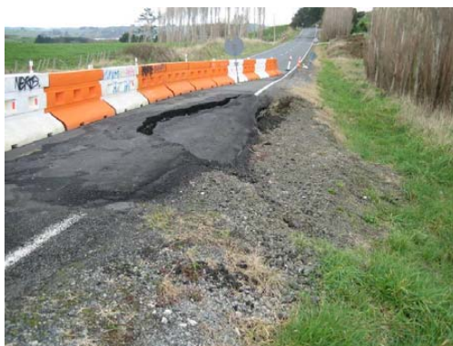
Figure 1: View of Wharehine Road showing collapse in Pavement
