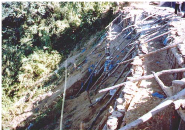
Figure 2: A photograph of damaged slope and temporary slope protection works by wooden piles
