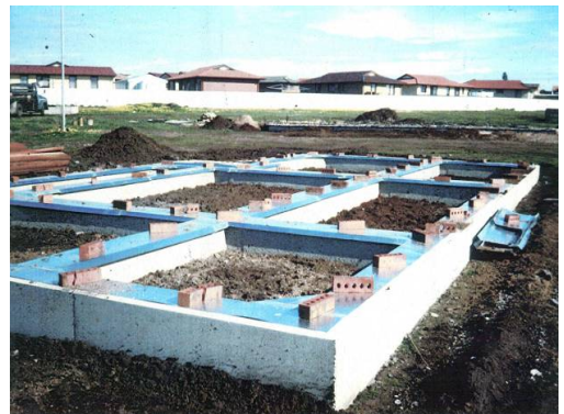
Figure 6: Gridded strip footing (for suspended flooring)
