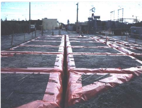
Figure 5: Gridded raft footing
