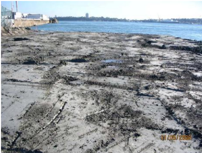
Figure 16: Completed mudcrete subgrade
