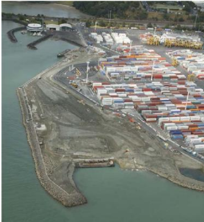
Figure 13: Fergusson Wharf reclamation
