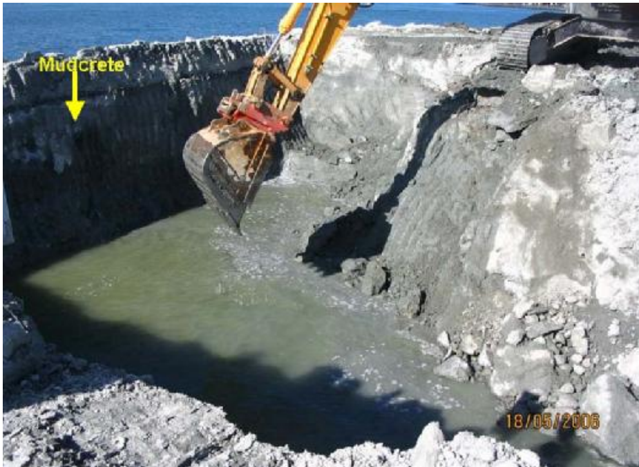
Figure 15: Trenching in mudcrete
