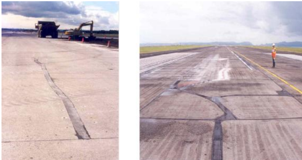
Figure 18: Fatigued slabs
