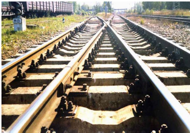
Figure 4: Railway sleepers built in 1989 of pre-stressed slag alkaline concrete, Moscow - St Petersburg railroad (Krivenko 2005).
