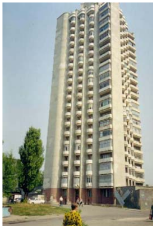
Figure 3: 24 storey residential building built in 1987-89 of slag alkaline concrete (Krivenko 2005).
