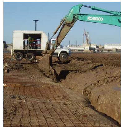
Fig. 8 - CPTu testing on top of barrier wall
