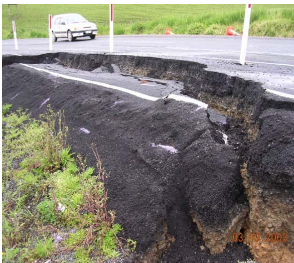
Figure 1 (left): A typical New Zealand road under slip. Figure 2 (right): The Colmix C1300 rig
