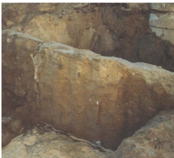
Figure 7: Overlapping columns creating cells.
