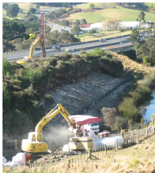
Figure 5: Installation of DSM columns at Okura.
