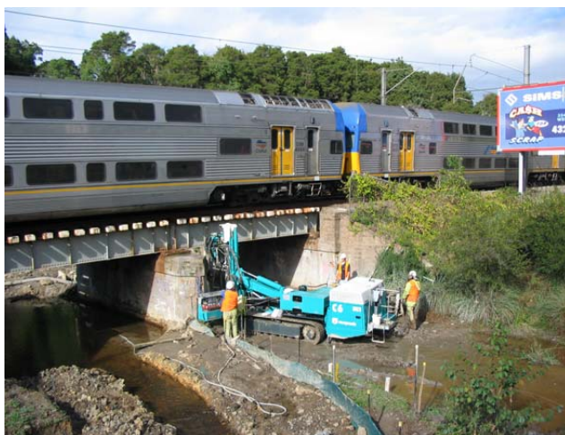
Figure 2: Previous bridge showing jet grout installation
