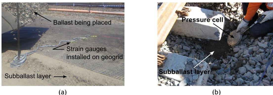
**Figure 5: Installation of (a) strain gauges and (b) pressure cells to monitor response of track substructure under repetitive wheel loads.**
