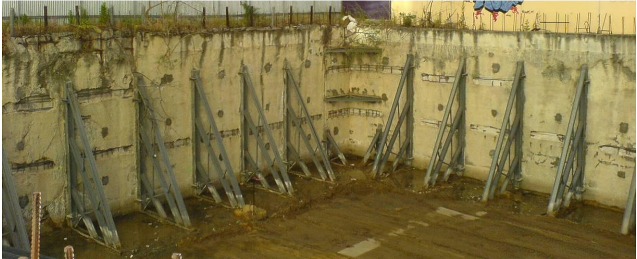
Figure 7. Steel struts supporting diaphragm walls; photograph taken after initial site cleanup
