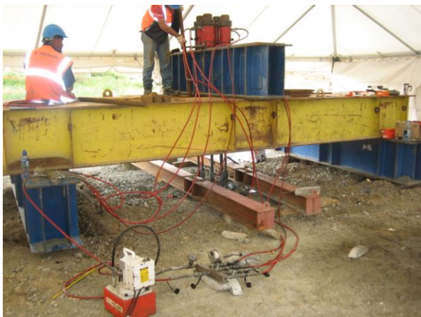
Figure 2: Pile test setup
