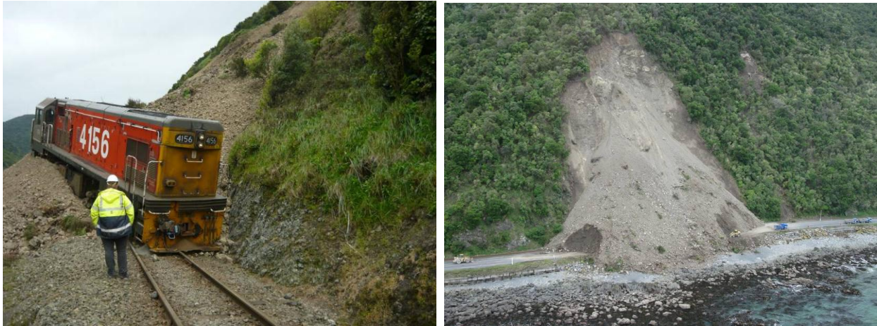
Figure 1: Recent landslides along the NZ rail corridor. Left: Palmerston Nth – Gisbourne Line (PNGL) near Woodville, North Island (Sept 2010). Right: Main North Line (MNL) south of Kaikoura, South Island (Sept 2010).
