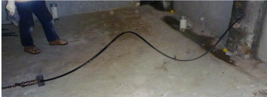
Figure 8: Removal of tendon using winch
