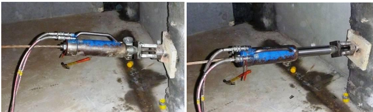
Figure 7: Hydraulic jacking of removable tendon
