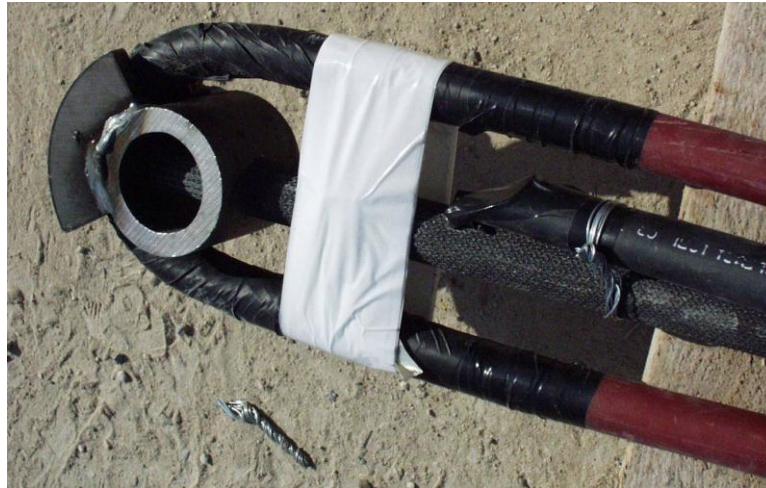
Figure 3: Saddle arrangement for Removable SBMA systems
