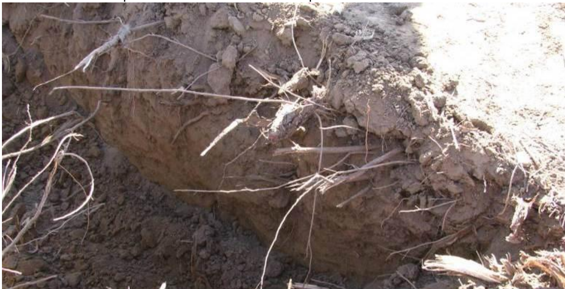
Plate 4 Typical Gilgai Cracked Soil & Root Zone
