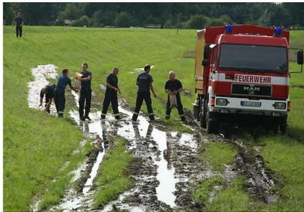
Figure 11. Softened levee toe
