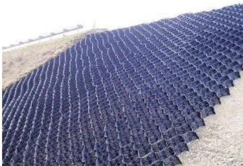
Figure 8. Installed geocells at a slope (RKL)
