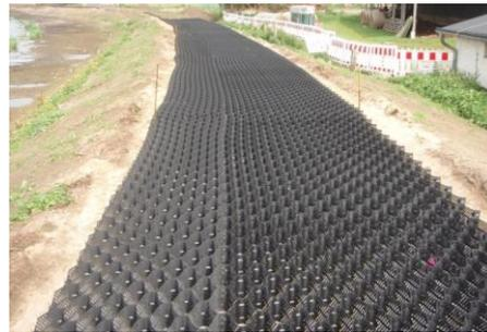
Figure 12. Geocells at the crest of an embankment
