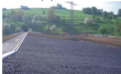
Figure 5. Open stone asphalt
