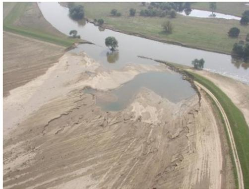
Figure 1. Levee failure at the river "Vereinigte Mulde" near Laußig in Germany, 2002 (Heyer 2007)
