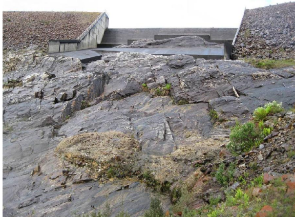
Plate 1: Unweathered foliated quartzite exposed in the spillway. Note the gravelly brown (basal till) remnants on the rock in the foreground.
