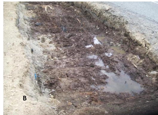
Figure 1. New railway embankment under construction (a) and peat exposed at the ground surface (b)
