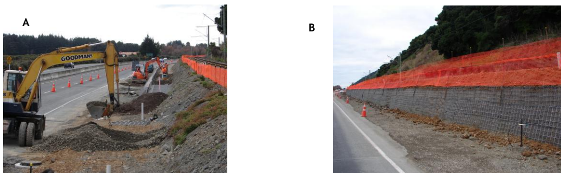
Figure 5. Terramesh Green walls during (a) and immediately after construction (b)
