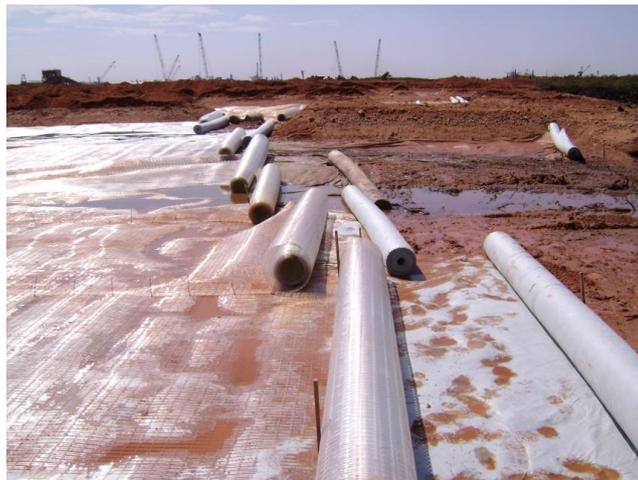
*Figure 3 Photograph of Basal Geogrid Reinforcement*
