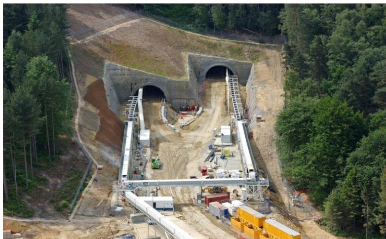
Figure 6 – North portal temporary soil nailed slopes
