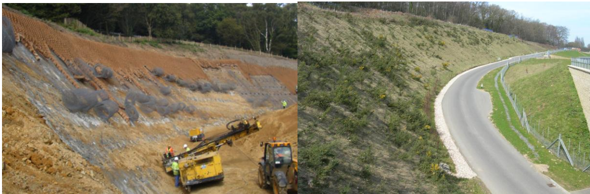
Figures 2 & 3 – Blackhanger Cutting 45° flexible facing during construction, and post construction
