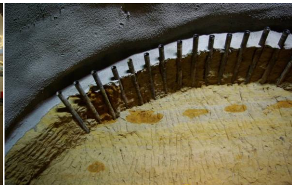
Figure 4, Typical canopy tube installation
