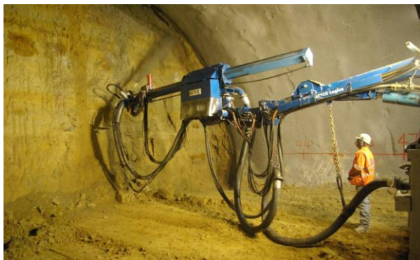
Figure 3, Primary lining application
