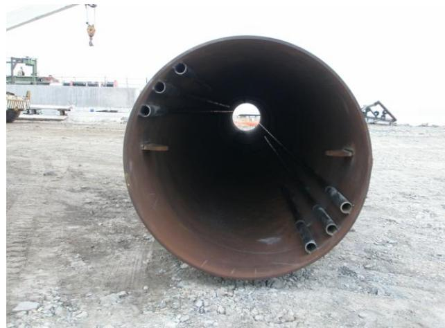
Figure 2. Telltale casings installed on test pile
