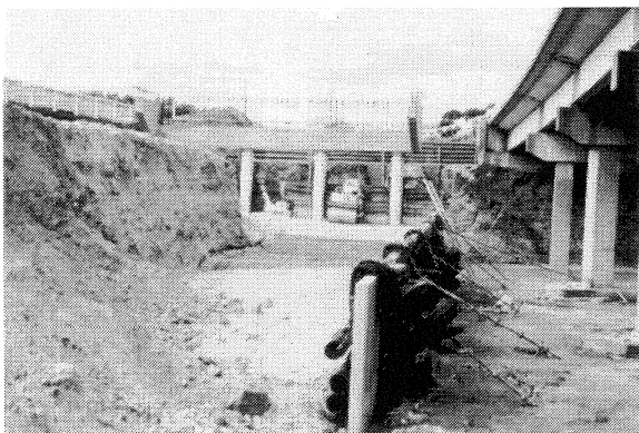
Figure 3. Abutments during backfilling.
