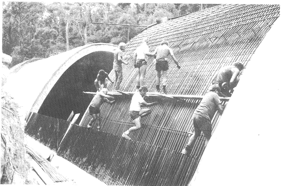
View showing reinforcement and size of culvert
