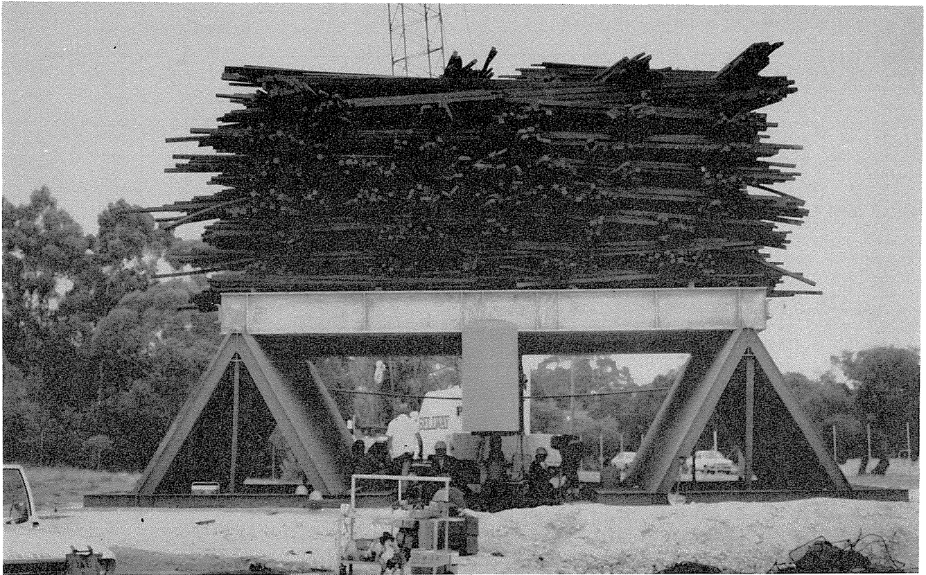
Figure 6 View of pile load test
