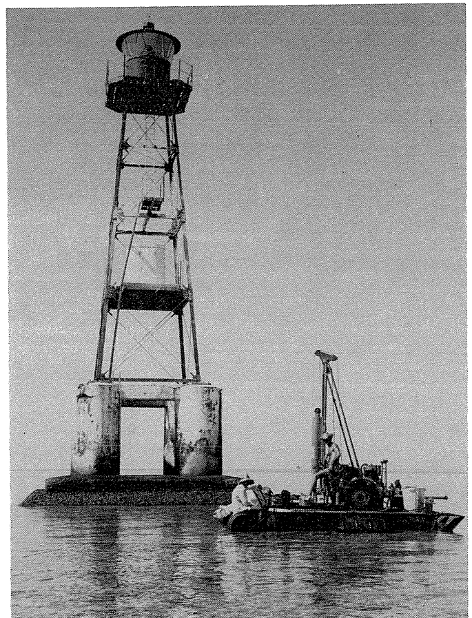
Fig. 2 Site investigation with the heavy dynamic probing technique for the foundation of a new lighthouse on Heath Reef (Area 1, Fig. 1)
