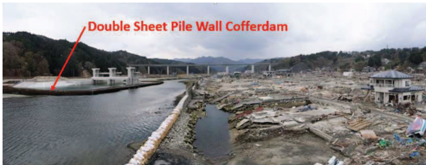
Figure 2. Tsunami-survived double sheet pile cofferdam in Yamada Town, Iwate Prefecture, Japan (Japan Press-in Association, both Figures 2 and 3)
