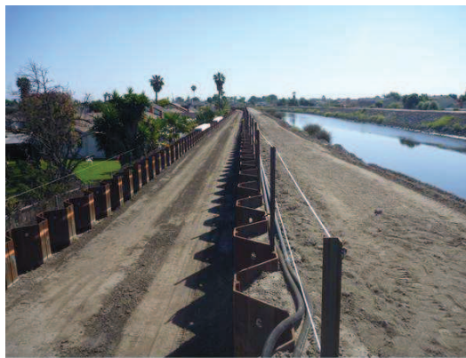
Figure 9. Completed double sheet pile walls
