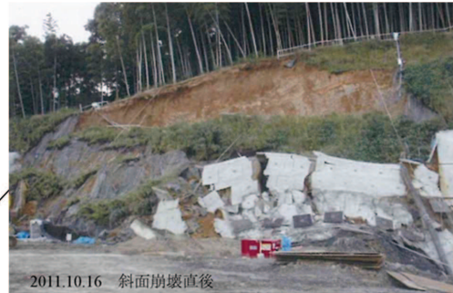
Photo 1. Collapse of slope A.
