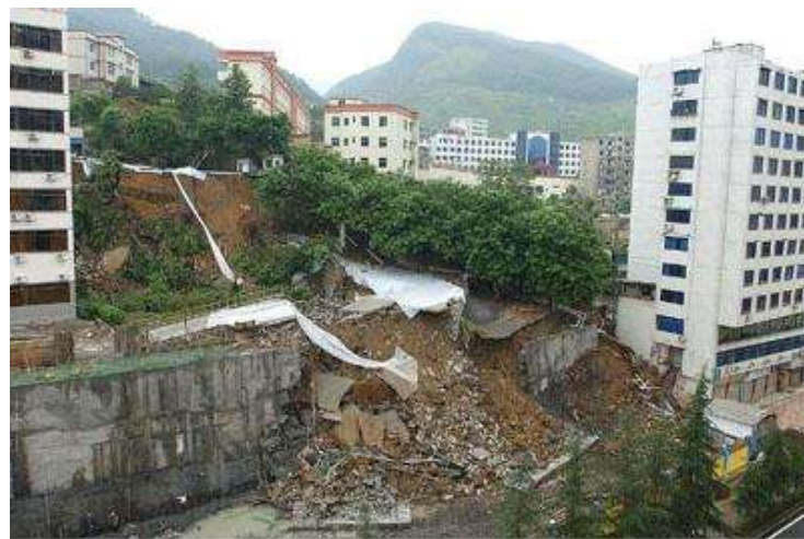
Fig. 12. Panoramic view of Wulong ‘5.8 Government Office Landslide’ in Chongqing, China
