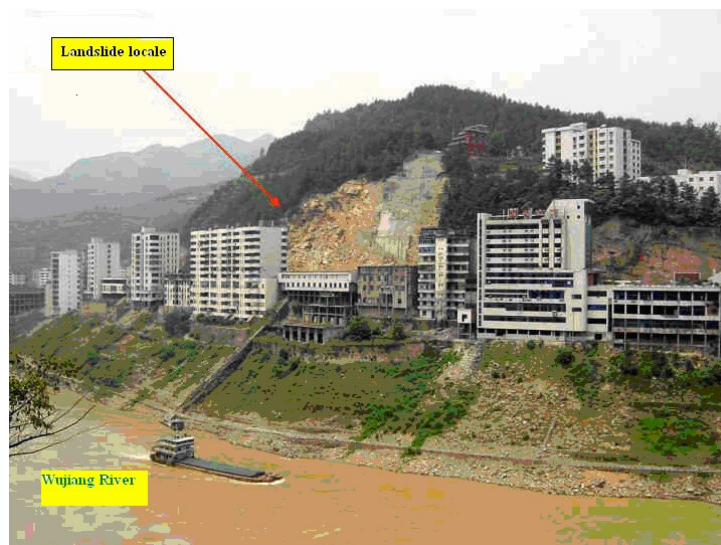
Fig. 1. Panoramic view of Wulong ‘1 May’ landslide area
